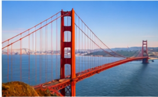
Golden Gate Bridge
